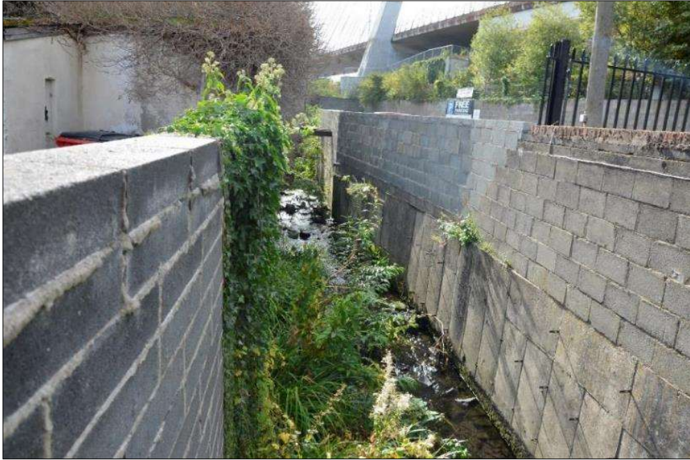
Plate 7.1 The heavily modified Slang River (site 1) at Dundrum Luas bridge, bounded by high retaining walls
